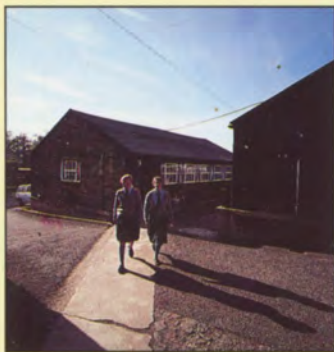
Two of the huts which will be demolished.
